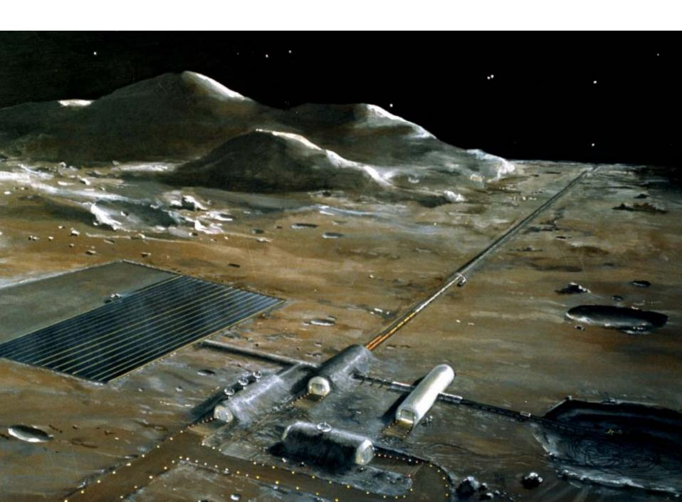
Rail guns (and gas guns) are simple but suffer from problems of low throughput and hypervelocity erosion
