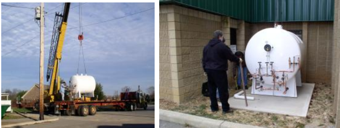
Figure 10. Left: Delivery of the leased 500-gal LN 2 tank. Right: Installation of the tank at the exterior wall of the dedicated MARS-LTB simulation laboratory. Subsequent to installation a safety fence with a locked gate was installed around the tank.
